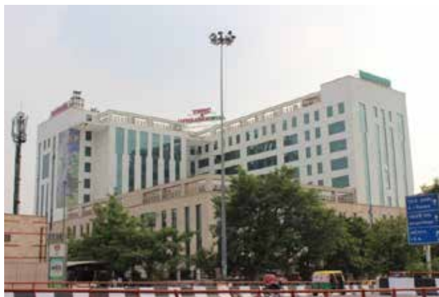
New emergency block
